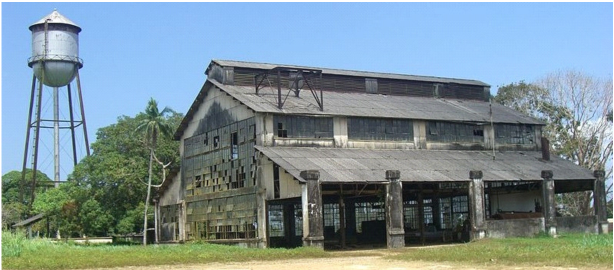
A Recent Photograph of the Abandoned Water Tower and Machine Shop.
